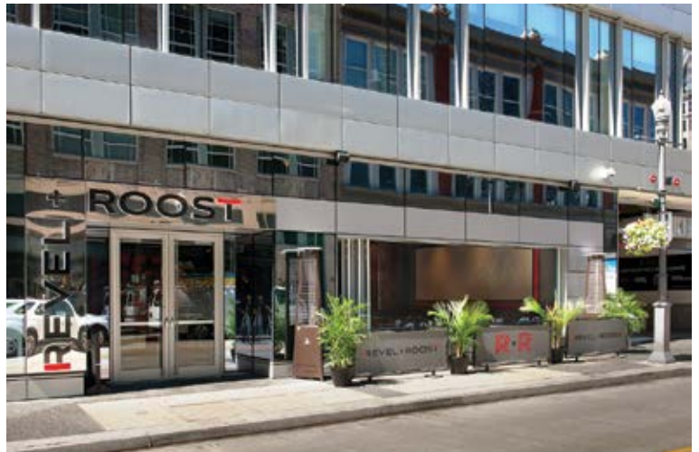
A folding aluminum window system was used in place of fixed storefront to bring the outdoors into Revel. Photo by Craig Thompson.
